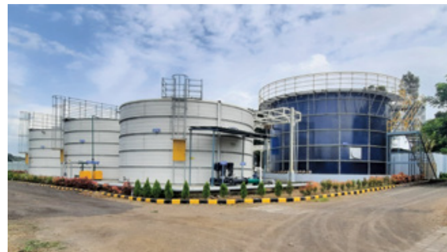
ETP and RO plant in factory
