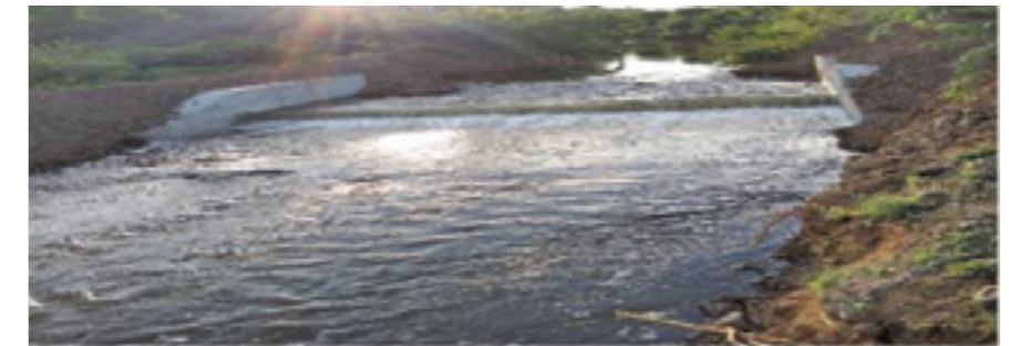
Cement dam at Chowdary wasti Khor
