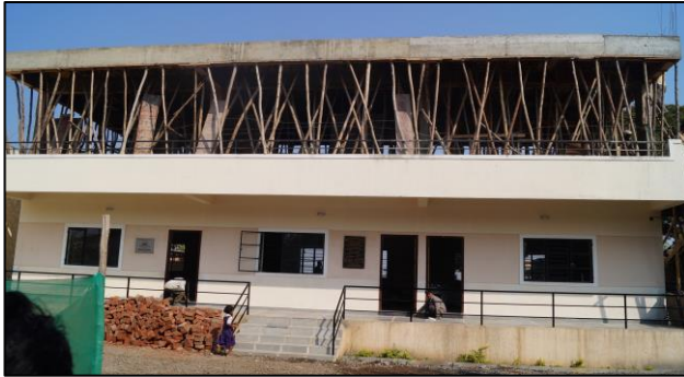
New Classrooms constructed for Bhandgaon School
